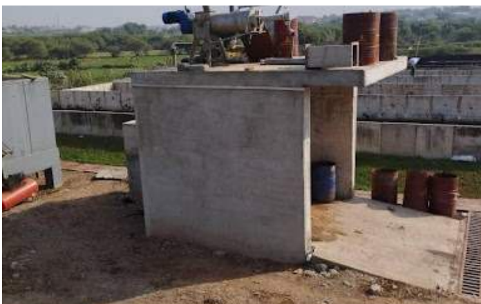
Screw press which is placed between the digester and drying beds
